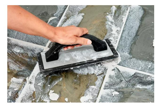
**Tip**: Don't worry about making this entirely neat. It's inevitable that some grout will get on the tiles during this process. Luckily the sealant you applied will protect the slate from permanent damage, and you will be able to remove it during the next step.
